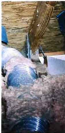
Roof to wall attachment
