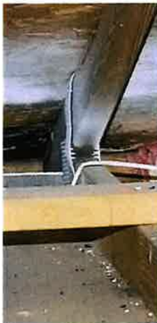
Roof to wall attachment
