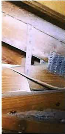
Roof to wall attachment
