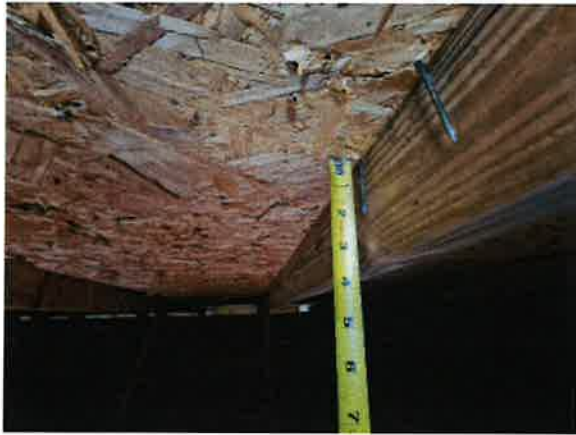
Deck to truss connection
